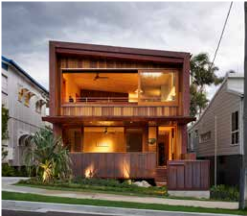
MOFFAT BEACH HOUSE RICHARD KIRK ARCHITECT
