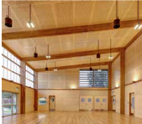
MATRAVILLE YOUTH & CULTURAL HALL SAM CRAWFORD ARCHITECTS
