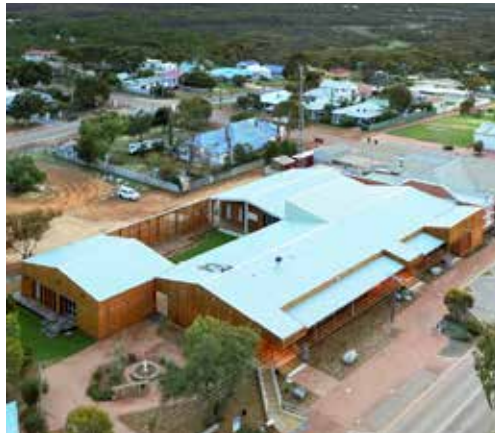
RAVENSTHORPE CULTURAL PRECINCT PETER HOBBS ARCHITECTS
